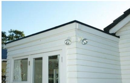
**Figure 4:** Bitumen membrane skillion roof
