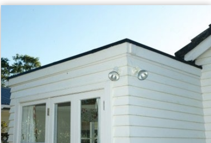
Figure 4: Bitumen membrane skillion roof
